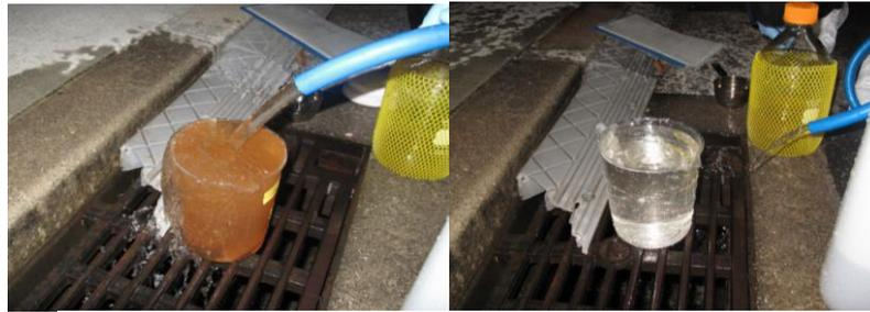
**Photo 2.** Pipe cleaning by conventional flushing.
